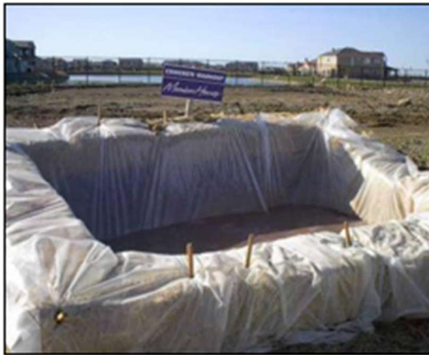
Plate 3-1 Typical concrete wash out areas
